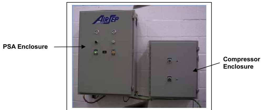
Figure 3.1: CENTROX Oxygen Concentrator
